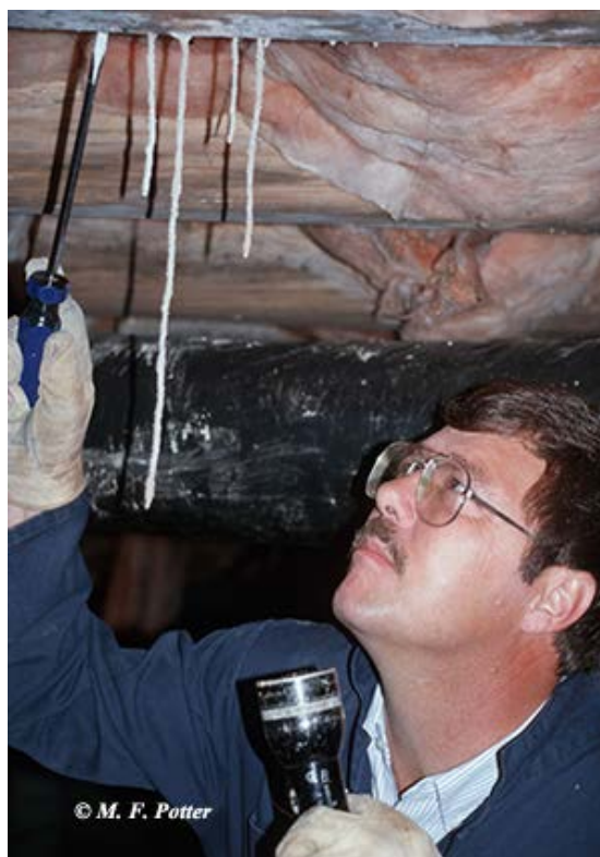
Fig. 9: Termite inspections and treatments are best accomplished by professionals.
