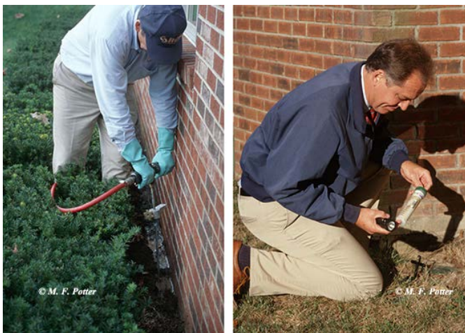
Fig. 8: Two treatment options for termites: liquid application (left), baiting (right)
